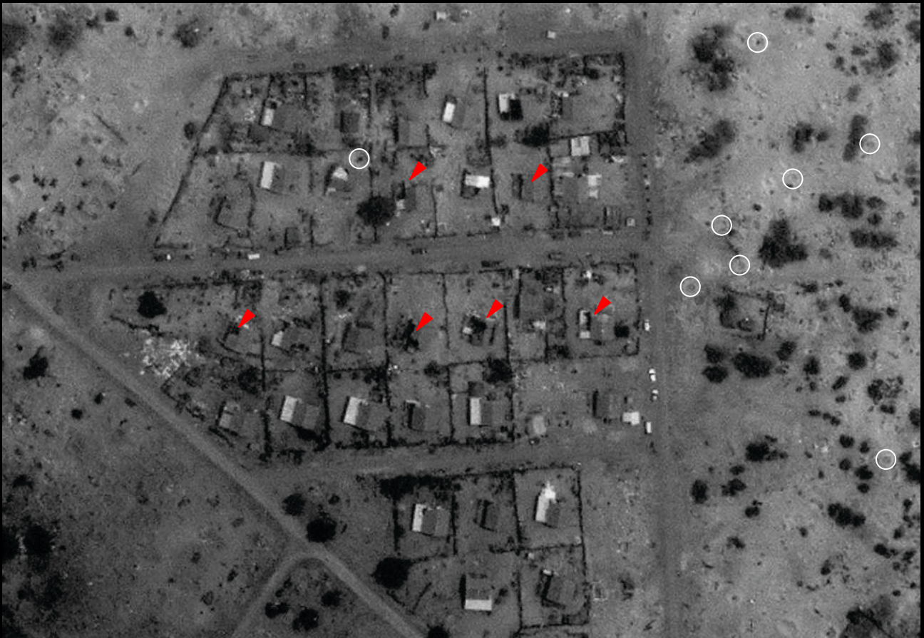
Figure 9.4-25: Damage to buildings due to mortar – See the qualitative differences in the damage pattern. House damaged by mortar shells have most of their roofs intact. Area Karaiyamullivaikal – Source: earth.google.com
